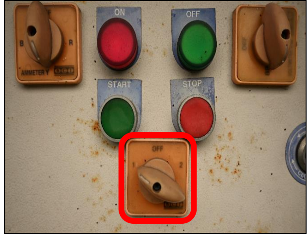
Fig. 36. The Chiller is set in AUTO-MODE condition (the switch is turned to the left for auto mode)
